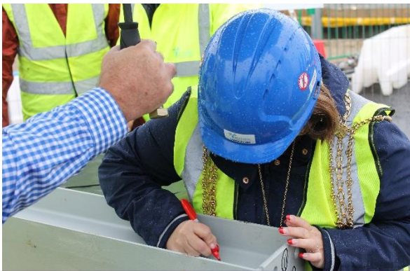
The Lord Mayor of Leeds signing the final beam of the Springwell Leeds, North site structure.
