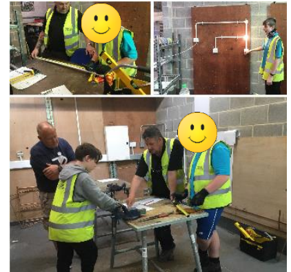
Our children learning some plumbing and electrical skills
